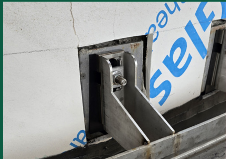
Molabolt Peg Anchor, Fairwater Campus Project, Cardiff – Advanced Bolting Solutions Limited
